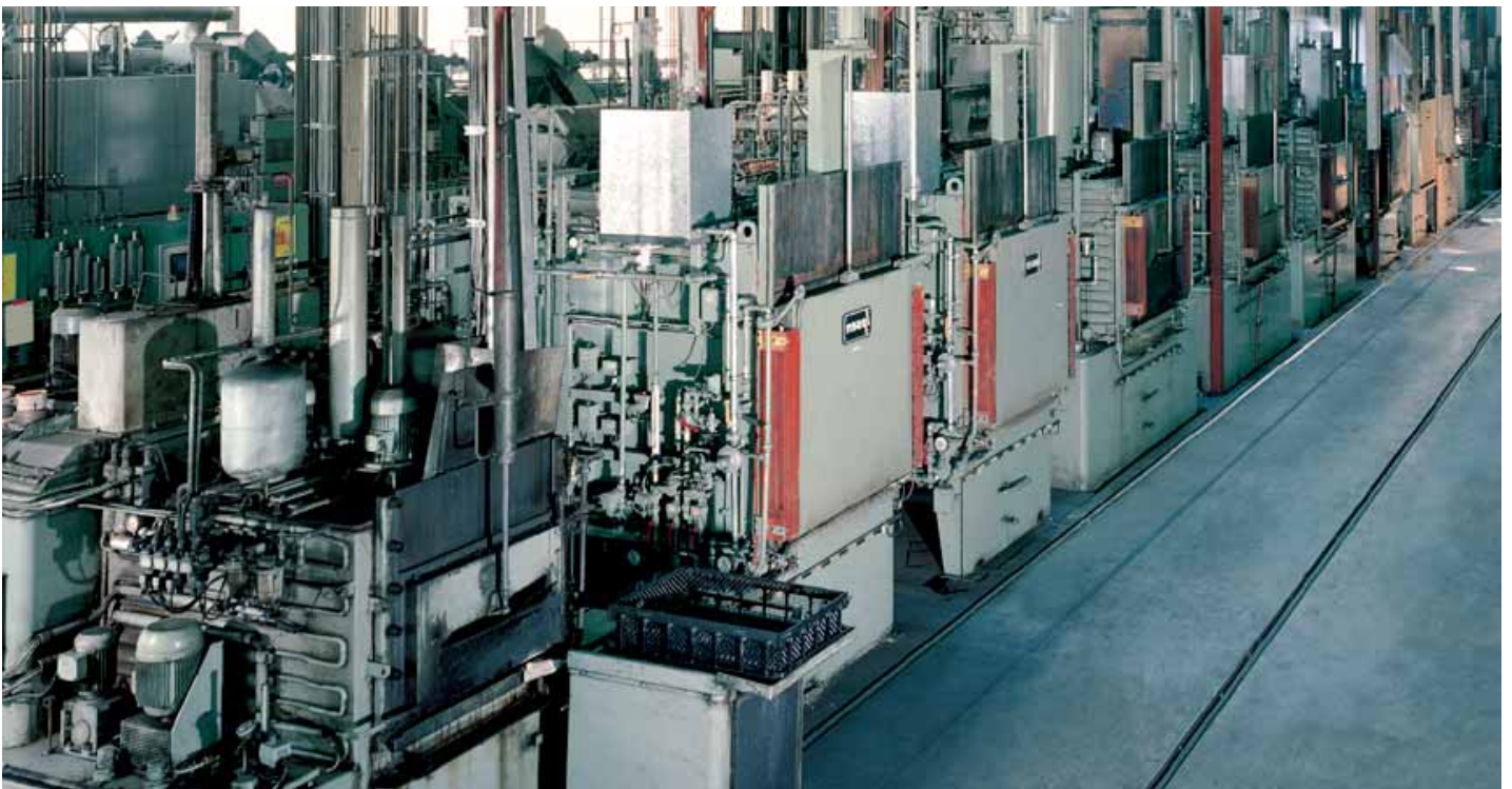
View into hardening shop with a row of sealed quench furnaces
