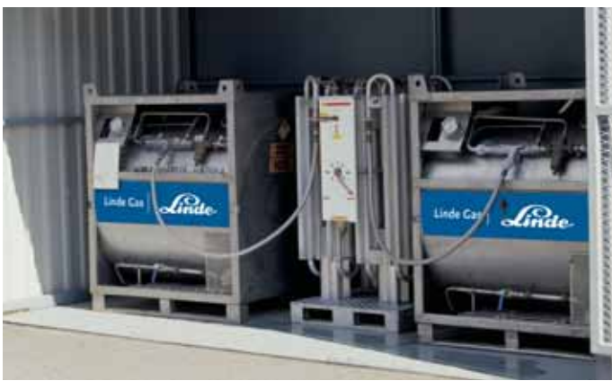
Figure 15: Liquid Nitrogen Stored in a Pallet Tank Holds Typically 600 Liters (300 Gallons) of LIN
