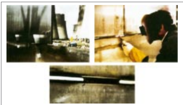
Fig. 11 FGD-flue gas absorber Welding of clad plates in position PC
